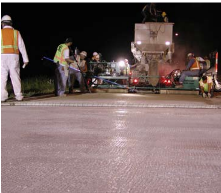
Above: Rapid setting concrete placement on Highway 99 ramp, Bakersfield.
