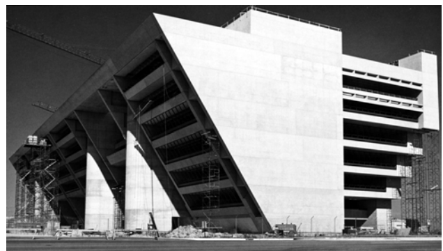
Fig. 4 – Dallas City hall during final stages of construction
