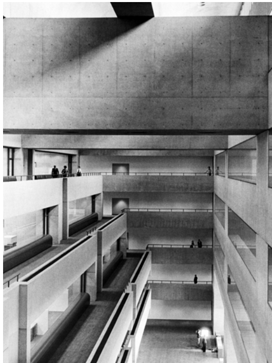
Fig. 7 – View of the cantilevered box beam
