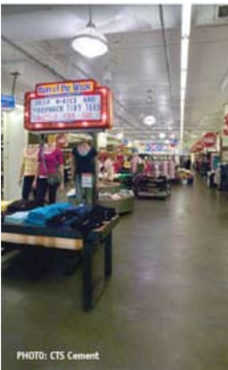
The Portland Ore., Old navy retail outlet required floors with minimal joints for improved appearance, and safer navigation. A light sandblast finish was completed before sealing the floor.
