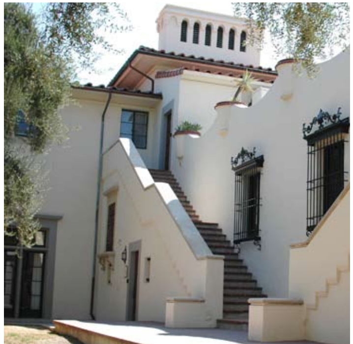
High-performance rapid-setting cement helped replace a number of badly weathered concrete stairways. Photos: CTS Cement Manufacturing Corp.
